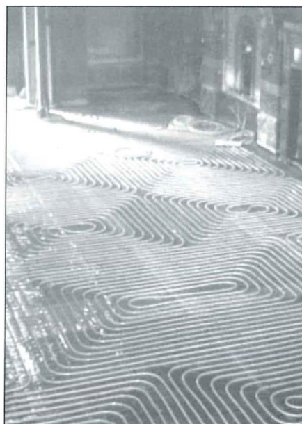
Figure 11 Double coil layout
