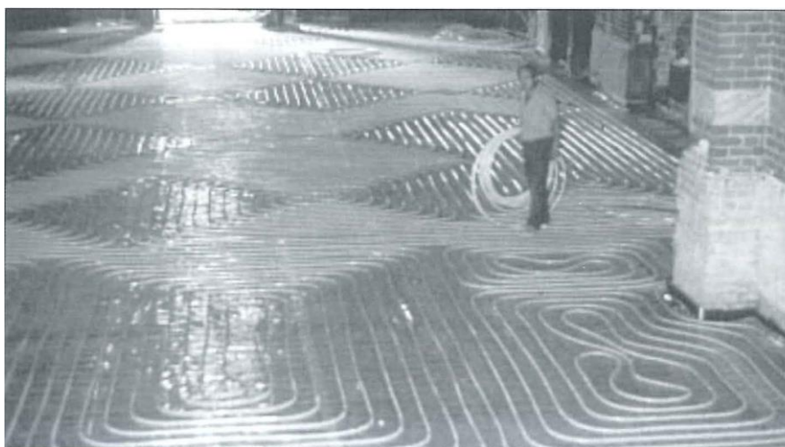
Figure 12 Spiral coil layout
