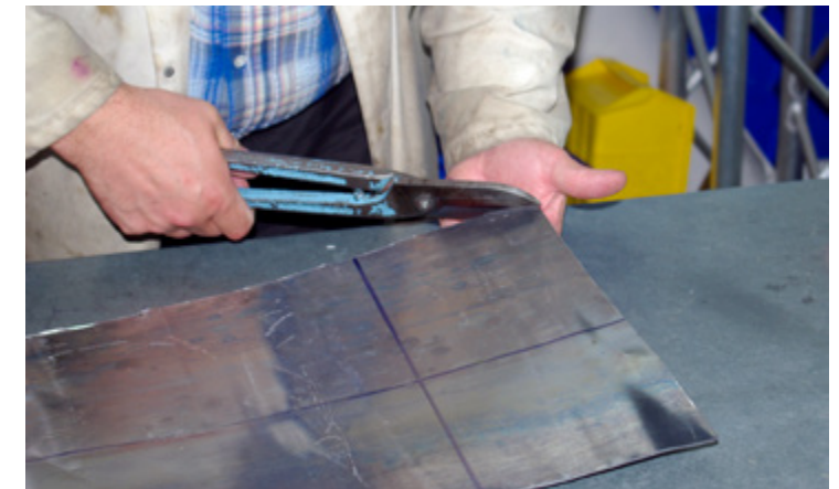
Step 1: Marking and trimming the lead
