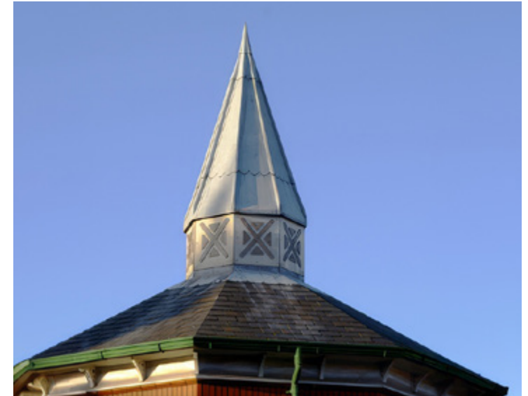
The effects of rain washing off the lead patina (Photo: Mike Maskrey)
