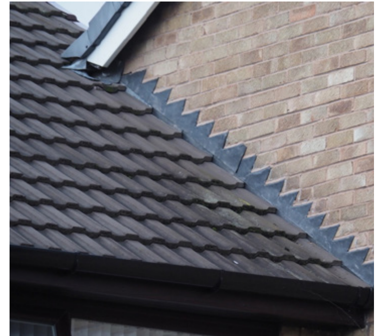
Step and cover flashing
