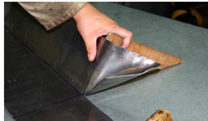
Bending the chimney line
