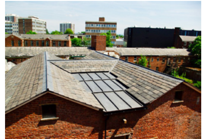
Traditional lead flat roofs
